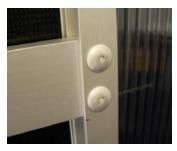
up using a pop rivet gun. The rivet head will stand proud of the Side Rail initially, but by compressing the rivet gun handles slowly while pushing down, the head of the rivet will become flush with the surface of the Side Rail. From this point on, the
