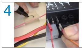
Mark any wires connected to this terminal (F) so that you can replace them in the correct position. Remove the wire from the terminal marked (F) on the Danfoss controller. Use insulation tape to protect the wire once it is disconnected from the terminal so it cannot contact other wires, electrical components or metal as shown in Section C, Step 5.
