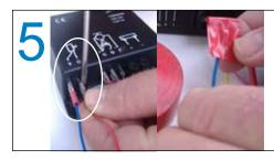
Disconnect any wires connected to the terminals marked (T) and (C) on the Danfoss controller. Use insulation tape to protect the wires once they are disconnected from the terminals marked (T) and (C) on the Danfoss controller so it cannot contact other wires, electrical components or metal. Fire could result if this wire is not insulated correctly. Always grip the crimped terminal, not the wire.
