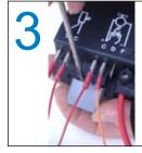
Locate the plastic fuse cover on the Danfoss controller - lever off with a screw driver.
